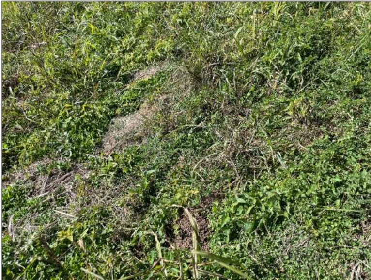
Photo 40, Point 28 Southeast Exterior Slope – Animal burrow.
