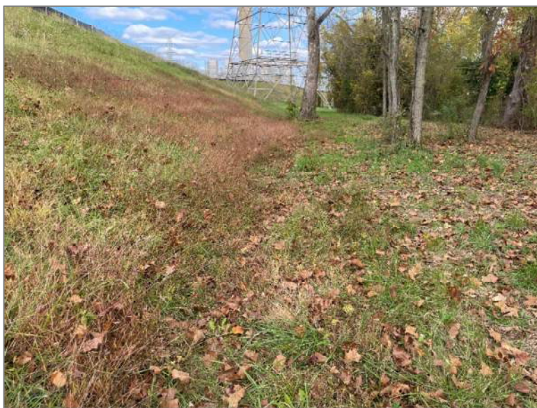
Photo 10, Point 7 Clearwater Pond – Southeast Exterior Slope – Drainage direction at toe unclear.
