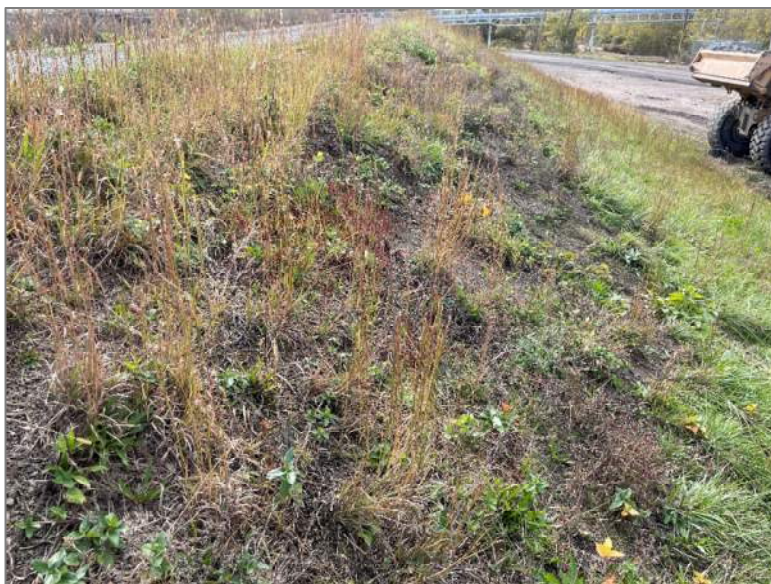
Photo 29, Point 19 Northwest Exterior Slope – Surface erosion, bare spots.
